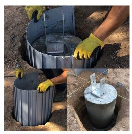
1. Reusable Form: With smooth side facing inside, can be used to cast concrete footings and columns. Once the concrete hardens, remove the Form-A-Tube® strips and save them for future use, making tubes of same or different diameters.
