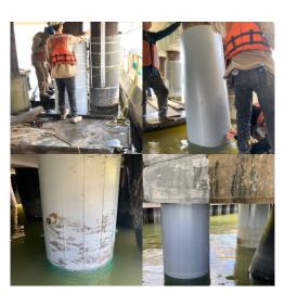
**2. Pile Encapsulation**: With the smooth side facing outside, can be wrapped around deteriorated piles or columns. The annular space is filled with concrete that interlocks with the ribs to create a long-lasting stayin-place form for repair and protection of pile or column.
