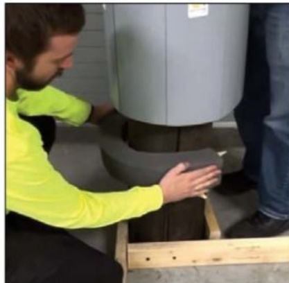
Secure the last strip with a mallet. Foam and a plastic skirt can prevent leaking grout from the annular space.
