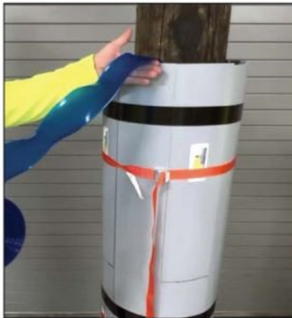
Ratchet strips are installed before the grout is placed using the tremie method. T profiles bond the tube to the grout.
