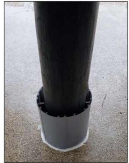
Ratchet strips are installed before the grout is placed using the tremie method. T profiles bond the tube to the grout.
