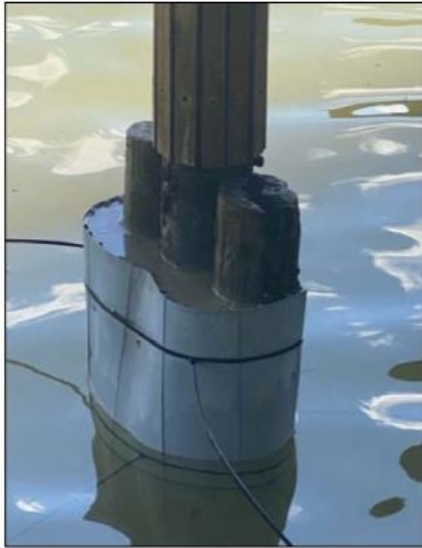
Form-A-Tube® strips can be used to create a tube of any shape.
