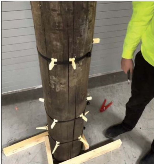
Spaces and skirt pins should be installed around a pile. Duct tape can be used to prevent the strips from sliding during handling and installation.
