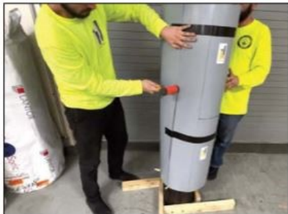
Secure the last strip with a mallet. Foam and a plastic skirt can prevent leaking grout from the annular space.
